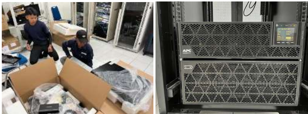
Gambar 3. 6 Instalasi UPS
